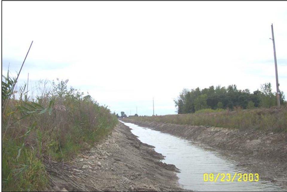
Maintenance of a natural buffer strip between spoils and reconstructed drain prior to drain bank stabilization.
